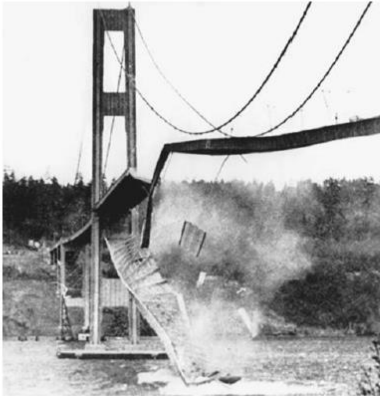
The Tacoma Narrows Bridge, November 7, 1940, a famous example of the phenomenon of resonance. The wind caused the bridge to begin to oscillate. Continued wind caused the amplitude of the oscillations to slowly increase until they tore the bridge apart. [Topham/The Image Works]
